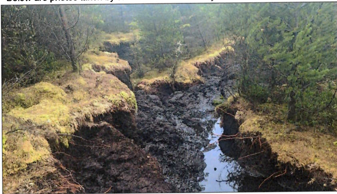
Plate 1 – Detached Peat Blocks at edge of failure zone
